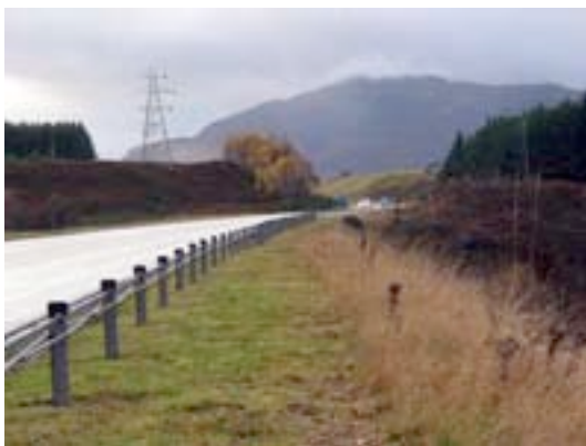
The A9 cuts through the hummocky terrain
